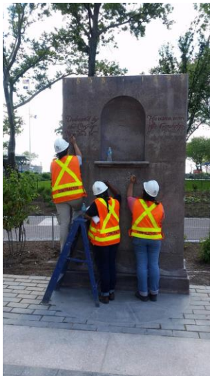
Conservators prime the letters before applying gold leaf - photo Jennifer Pont, Jablonski Building Conservation, Inc
