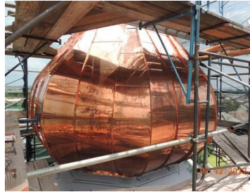
new dome with copper cladding
