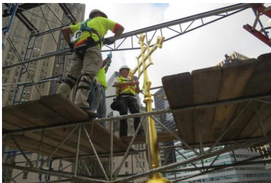
Re-installing the finial, photo Gilders' Studio, Inc.
