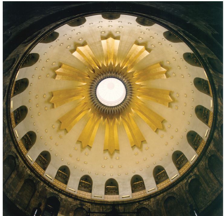
Above, at The Church of the Holy Sepulchre in Jerusalem, The Gilders’ Studio applied a linear textured pattern to the main rays, which were gilded with 23-karat gold leaf as were the stars and rings above it. The team also restored the circa 1869 gilding on the balustrades with 23-karat and 12-karat gold leaf.
